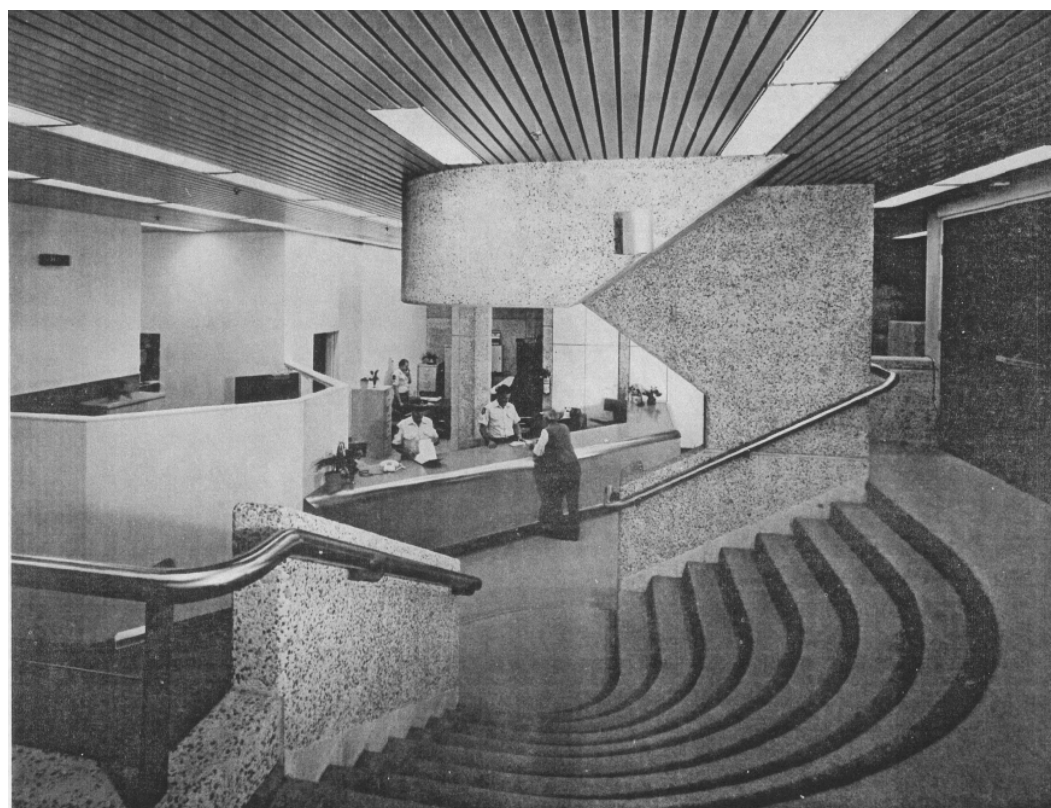
Figure 4.10 Public foyer of the Newcastle Police Centre photographed soon after construction. GAB Newsletter
