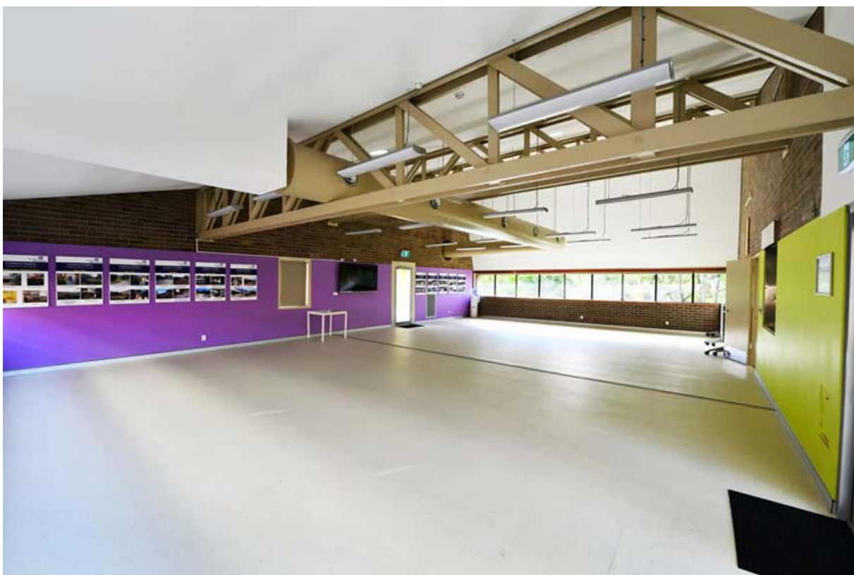
Figure 4.7 Hall at Keelong after refurbishment. Features such as the trusses and air conditioning ducts have been retained.
