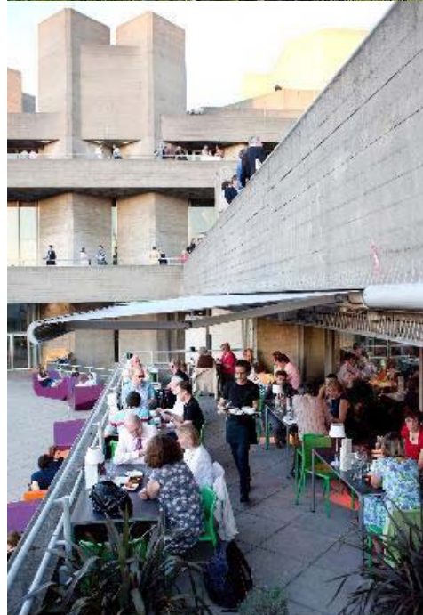
Figure 8.1 Landscaping upgrade to the terraces of the National Theatre on the Southbank in London. www.gardenbuilders.co.uk/p/5225/royal-national-theatre-garden
