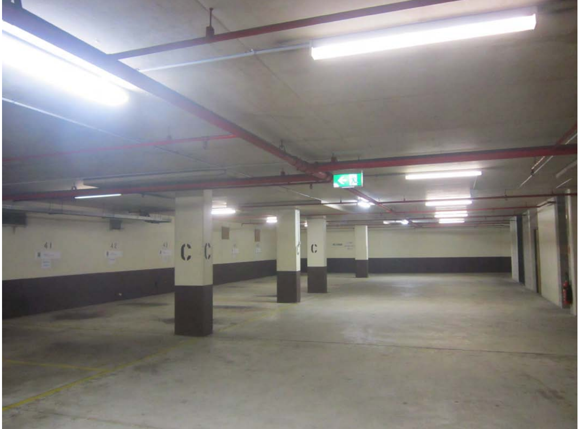
Figure 3.50 View of the car parking level C Photo: Noni Boyd, 2017
