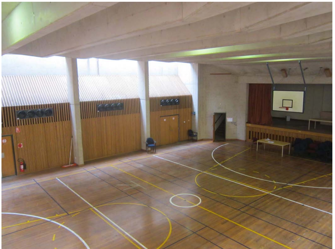
Figure 3.39 Multi-purpose hall. Photo: Noni Boyd, 2017
