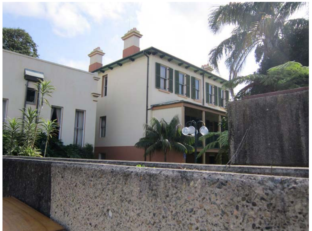
Figure 3.26 Details of the wall/planter box showing the exposed aggregate to the concrete. Photo: Noni Boyd, March 2016
