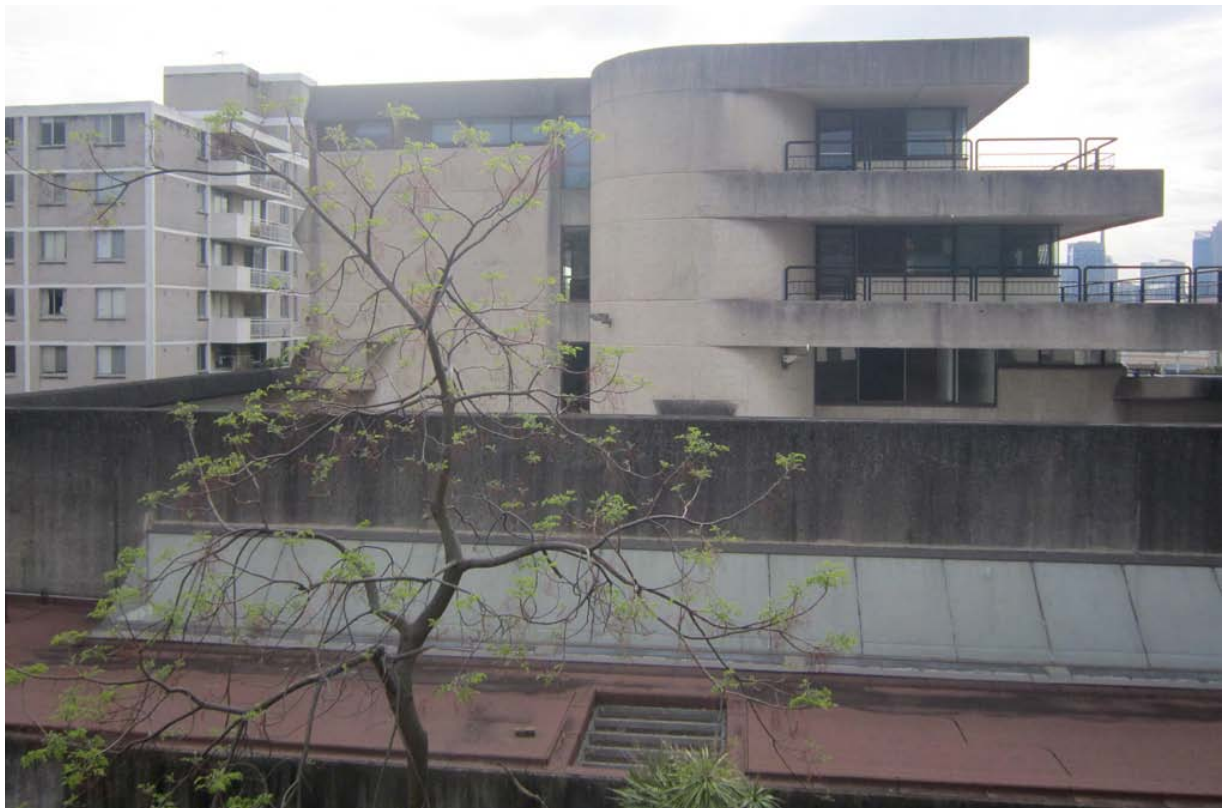
Figure 3.18 View from the first floor of the residence showing the staggered terraces and the lower scale of the MRC in relation to the apartment buildings beyond. Photo: Noni Boyd, 2017
