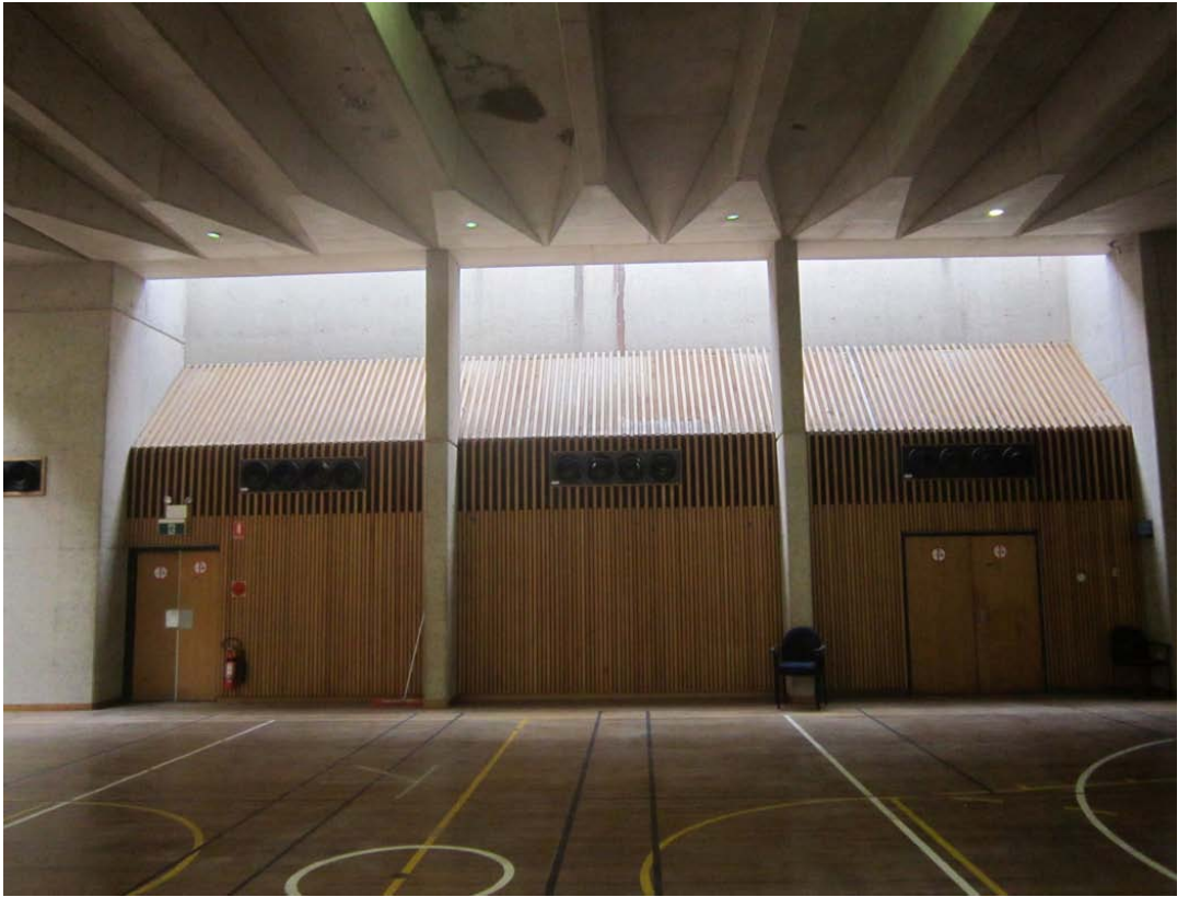
Figure 3.40 Multi-purpose hall as it appears today Photo: Noni Boyd, 2017
