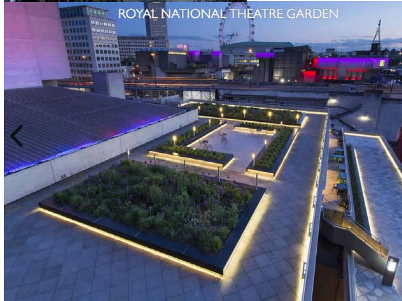
Figure 8.3 Night time view showing the new lighting scheme to the Royal National Theatre Garden. www.gardenbuilders.co.uk/p/5225/royal-national-theatre-garden
